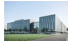
WORK'IN PARK 22 125 m 2 Gerland
